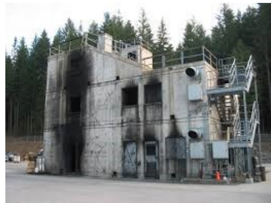
Figure 5. Firefighting training structure that uses clean propane gas
